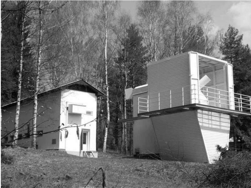
*Figure 1:* The HSFA2 telescope is located in a new part of the Ondřejov Observatory, surrounded by forest at altitude of 500 m above sea level. To the right is the coelostat tower, to the left the telescope. The spectrograph pavilion is on the first floor and the controlling room in the basement.
